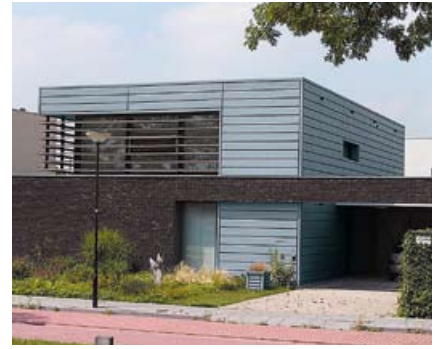
Private Residence, Empel, Netherlands
