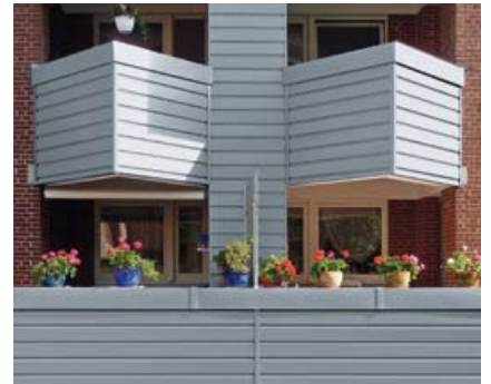
Multiple Dwelling, Neumünster, Germany
