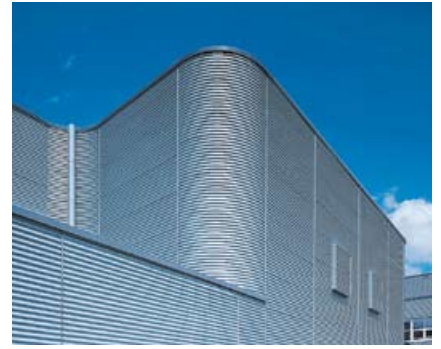
Multisport Complex, Walferdange, Luxembourg
