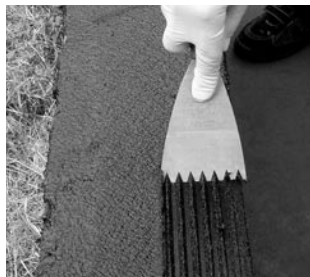
Fig. 5: Apply Enkolit® with notched trowel
