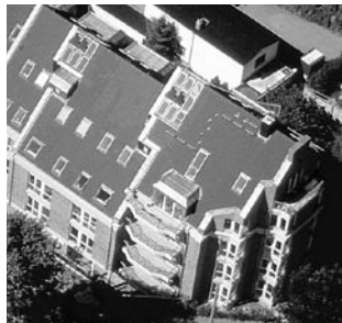
Fig. 31: Attic – cornice copings
