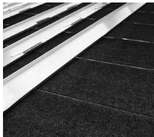
Fig. 9: Structured underlay, installation above wooden sheathing
