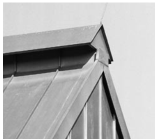
Fig. 17: Flush ridge termination on verge, high design
