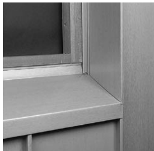
Fig. 26: Jamb on lateral connection windowsill coping
