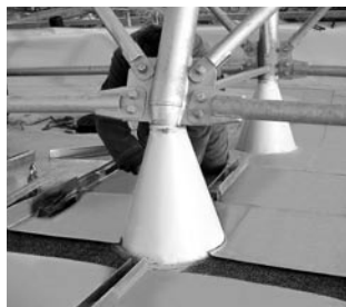
Fig. 7: Roof area with many penetrations
