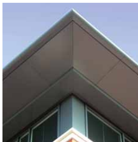
Stepped Interlocking Panels with bullnose fascia and internal gutter system.
